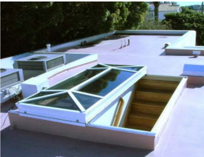
Location: Privet Residence, Manhattan Beach, Ca. Contractor: Sky-Tech Glazing Systems Description: One 4' x 8' Electrical Rolling Skylight.
