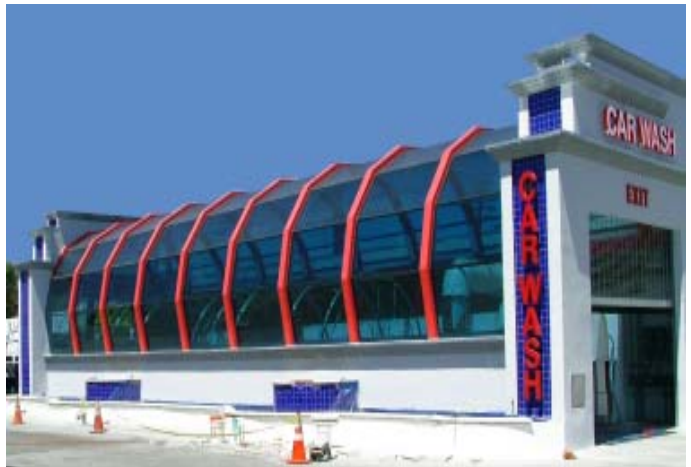
Location: Chevron Car Wash, Canoga Park, Ca. Architect: Leslie Lippich Architect Contractor: J.V.H Enterprises, Inc. Description: One 34' x 71' Segmented Half Barrel Vault
