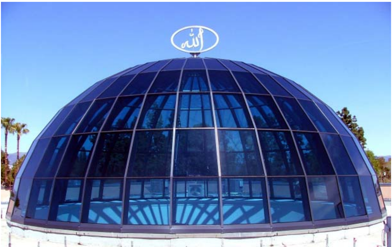
Location: MTO Shahmaghsoudi, Reseda, Ca Architect: GA. Architecture and Planning Contractor: Del Amo Construction Description: One 45' Diameter 20' Tall Segmented Dome
