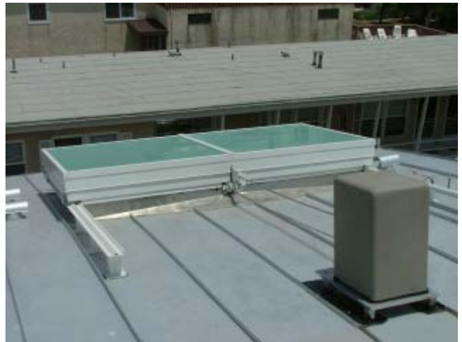
Location: Privet Residence, Hermosa Beach, Ca. Contractor: Baldwin Construction Description: One 5' x 12' Electrical Rolling Skylight.
