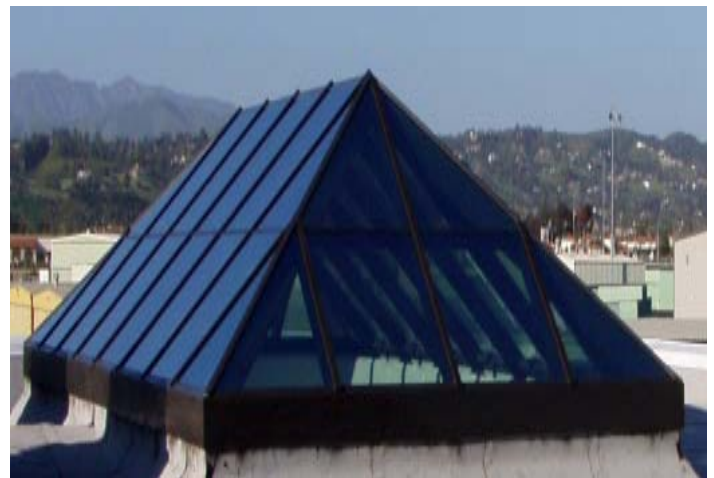
Location: Ventura Fire & Police Head Quarters, Ventura, Ca. Architect: Martinez Architects Contractor: Century Construction Description: One 14' x 27' Double Hip & Ridge Skylight.
