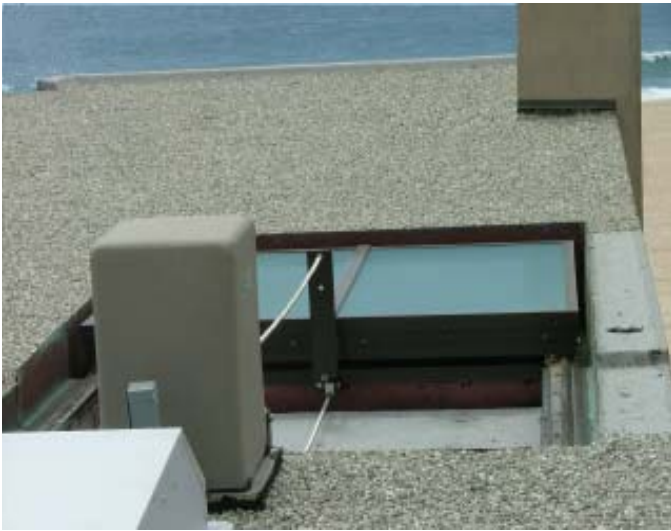
Location: Privet Residence, Hermosa Beach, Ca. Contractor: Baldwin Construction Description: One 4' x 6' Electrical Rolling Skylight.
