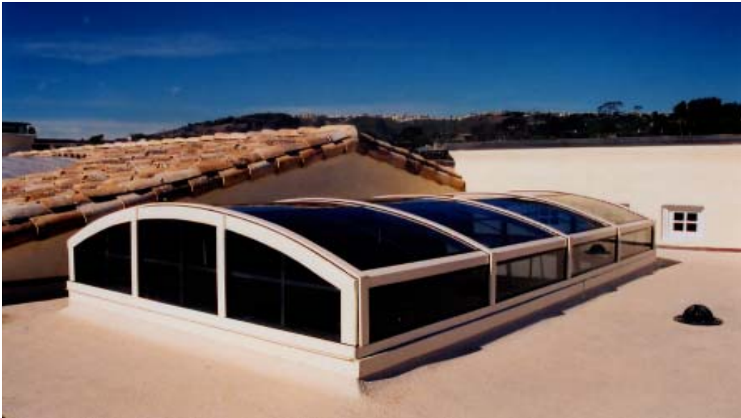
Location: Private Residents, Monarch Bay Dana Point, Ca. Contractor: Brock Lyster Construction Description: One 8' x 16' Barrel Vault Skylight.
