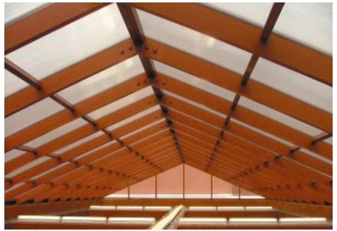
Location: Gabrielino High School, San Gabriel, Ca. Architect: Thomas Blurock Architect Contractor: Haselden Construction Description: One 32' x 95' Gable Ridge Skylight
