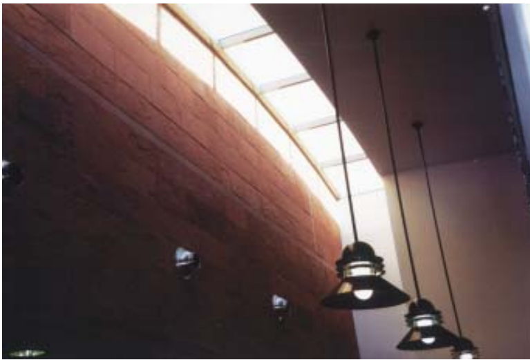
Location: Amtrak Station Bakersfield, Ca. Architect: Ordiz Melby Architects. Contractor: Colombo Construction Company Inc. Description: One 32' Radius Skylight, One 4' x 4' x 95' Ridge Lite.
