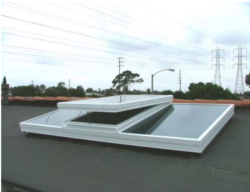
Location: Private Residents, Huntinton Beach, Ca. Contractor: Sky-Tech Glazing Systems Description: One 4' x 8' Flat Glass Skylight with Operable Bay.
