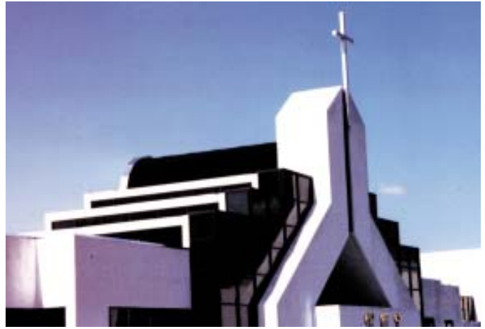
Location: Torrance First Presbyterian Church Torrance, Ca. Architect: Clean World Engineering, Inc. Contractor: John Kong Construction Description: One 24' x 12' Segmented Half Barrel Vault
