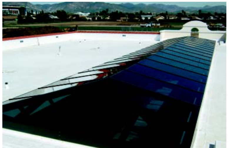
Location: San Fernando Mausoleum , Mission Hills, Ca. Architect: JST Architects Contractor: Carrier Mausoleums Construction USA, Inc Description: One 15' x 63' Hip&Ridge Skylight.
