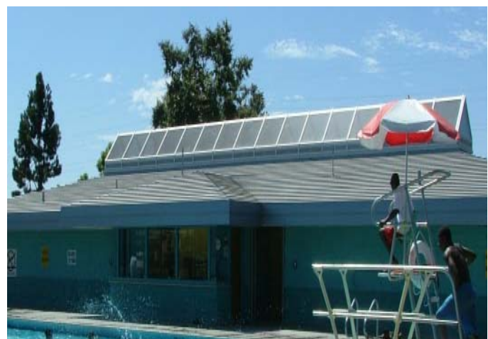
Location: Helen Keller Swimming Pool, Los Angeles, CA. Architect: Rachlin Architects Contractor: Mackone Development, inc Description: One 64' X 6' Gable Ridge With Louvers One 32' x 2' Gable Ridge With Louvers.
