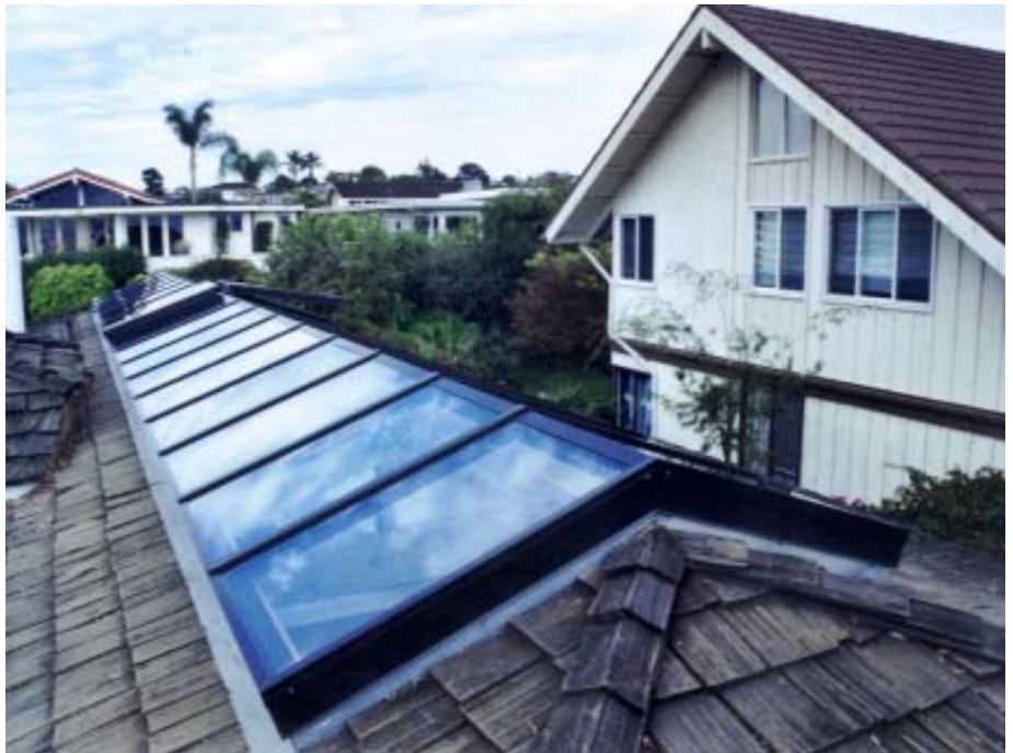
Location: Privet Residence, Corona Del Mar, Ca. Contractor: Sky-Tech Glazing Systems Description: One 45' x 4' x 4' Ridge Light Skylight With 2 Electrical Operable Bays
