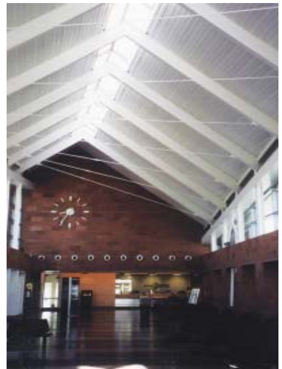
Location: Amtrak Station Bakersfield, Ca. Architect: Ordiz Melby Architects. Contractor: Colombo Construction Company Inc. Description: One 32' Radius Skylight, One 4' x 4' x 95' Ridge Lite.
