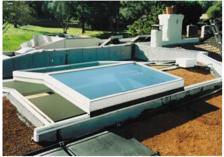
Location: Gomberg Residents Laguna Niguel, Ca. Contractor: C. F. Chicchetti Description: One 10' x 6' x 6' Electrical motorized ridge light
