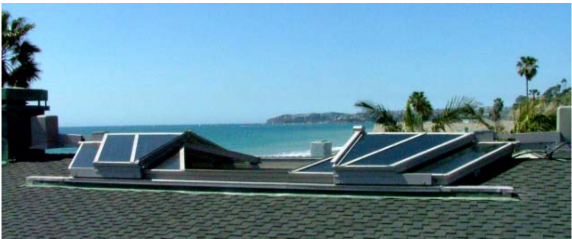
Location: Privet Residence, Manhattan Beach, Ca. Contractor: Sky-Tech Glazing Systems Description: One 10' x 30' Bi- Parting Electrical Rolling Skylights over Stationary Skylights.
